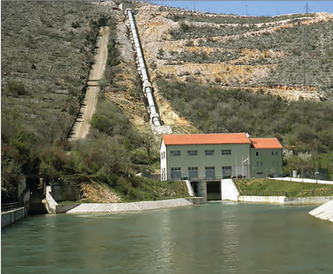
Figure 2.33 HPP Mostarsko blato, 60 MW, in operation since 2010
