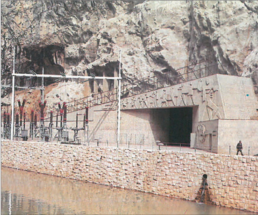
Picture 2.21 HPP Rama in operation since 1968, entrance to the machine room
