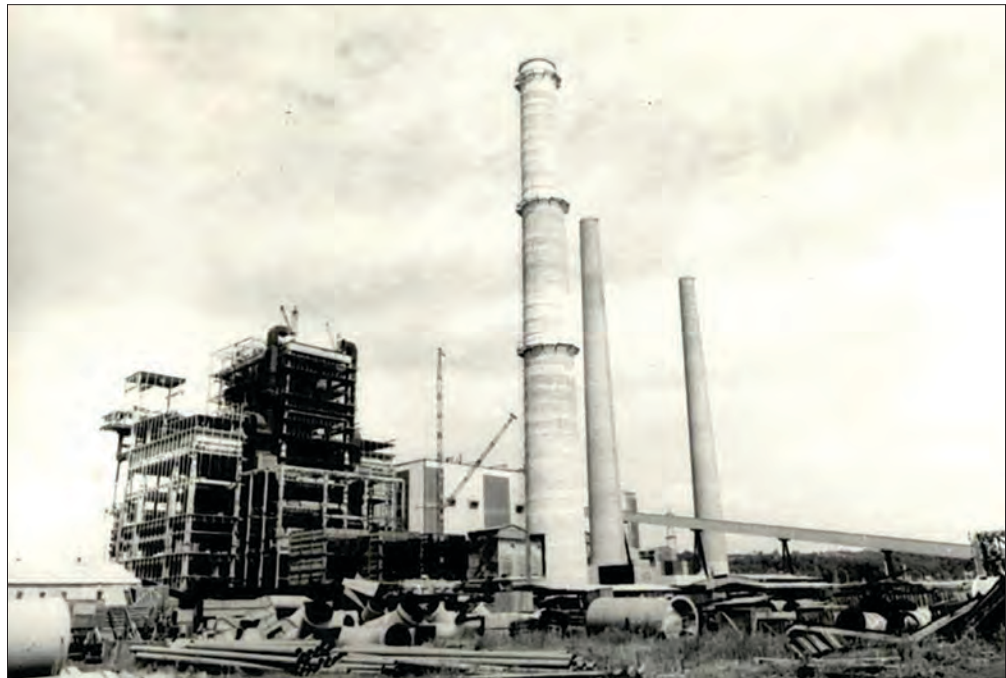
Figure 2.24 TPP Tuzla, III stage, 1971
