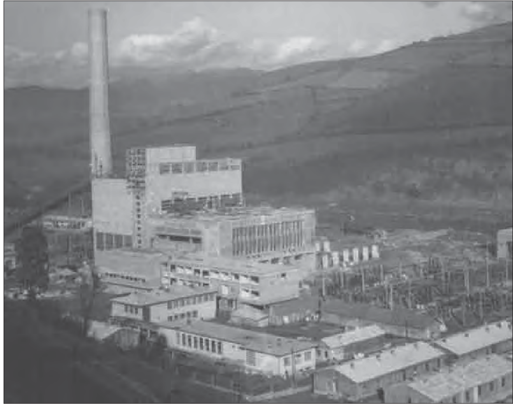
Figure 2.19 TPP Kakanj, Construction of Stage I (blocks 1 and 2), each 32 MW (1954–1956)
