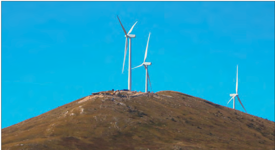
Figure 2.36 WF Jelovača, 36 MW, in operation since the beginning of 2019
