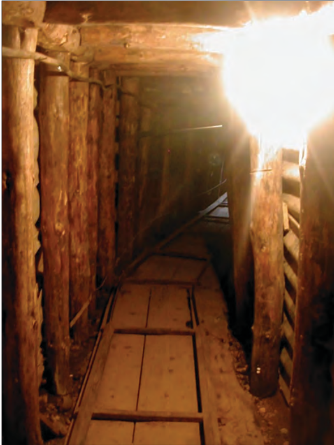
Figure 2.30 Rescue tunnel (35 kV cable installed)
