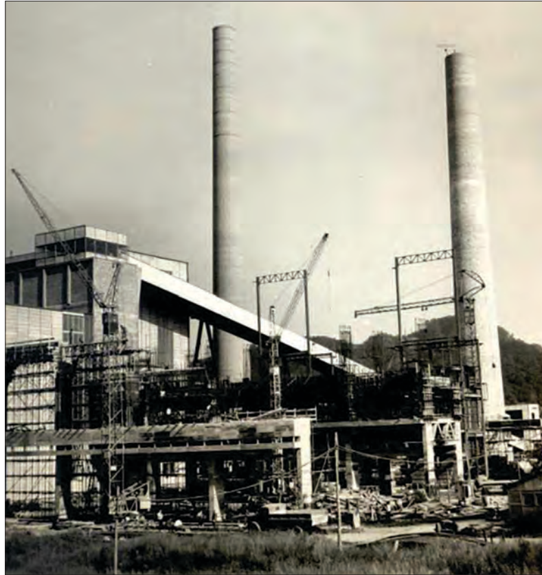
Figure 2.23 TPP Tuzla, Construction of the II stage, 1966
