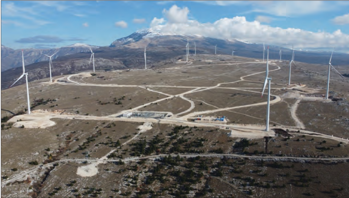
Figure 2.37 WF Podveležje, 48 MW in operation since 2021
