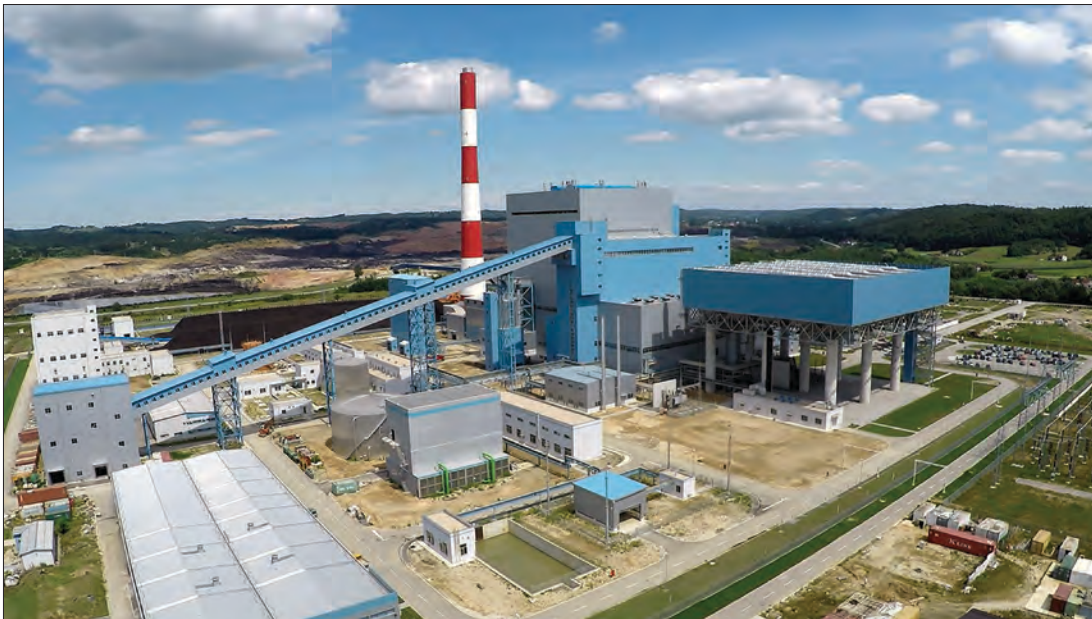
Figure 2.34 TPP Stanari, 300 MW, in operation since 2016
